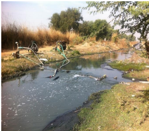
Figure 1. Water Pumps along the Dravyavati river to draw water for irrigation.
