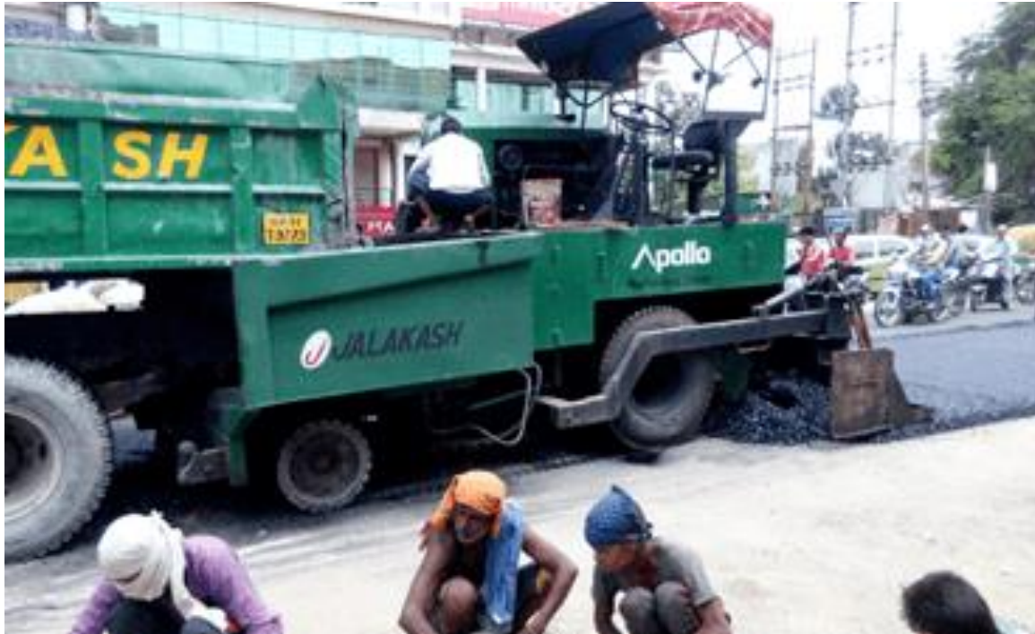
Figure 12. Mechanical paver is being used to spread the bitumen macadam.
