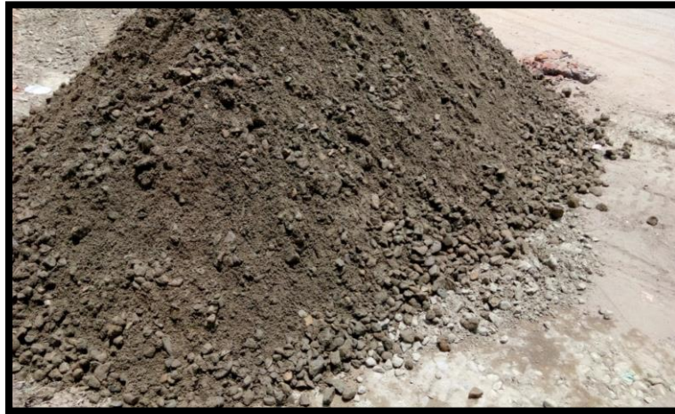
Figure 8. Water mix macadam used at the construction site
