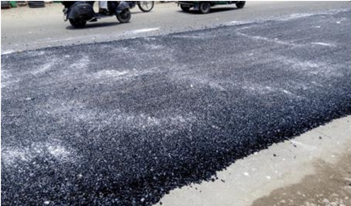
Figure 4. First layer Of Bituminous Macadam
