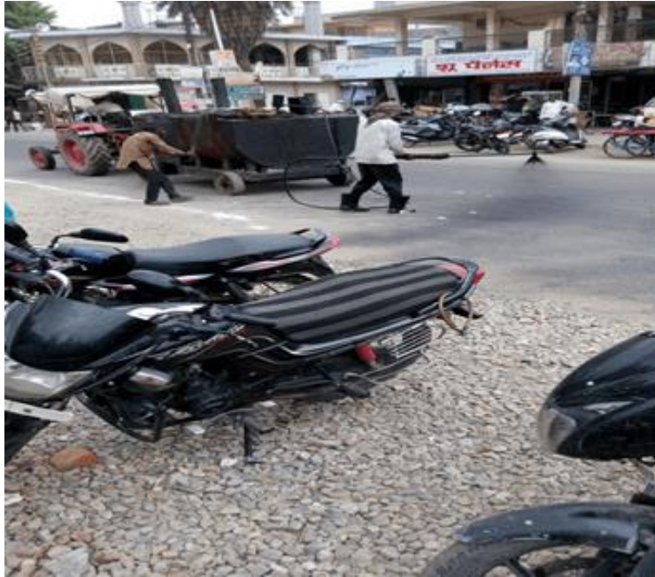
Figure 9. A tack coat is being applied before spreading the bitumen macadam on the pavement surface.
