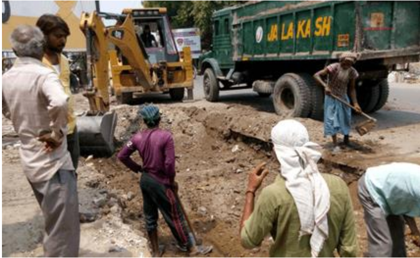
Figure 6. Excavation being carried out at the site
