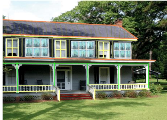
Figure 13. Green Building with plants, glass block and chimney
